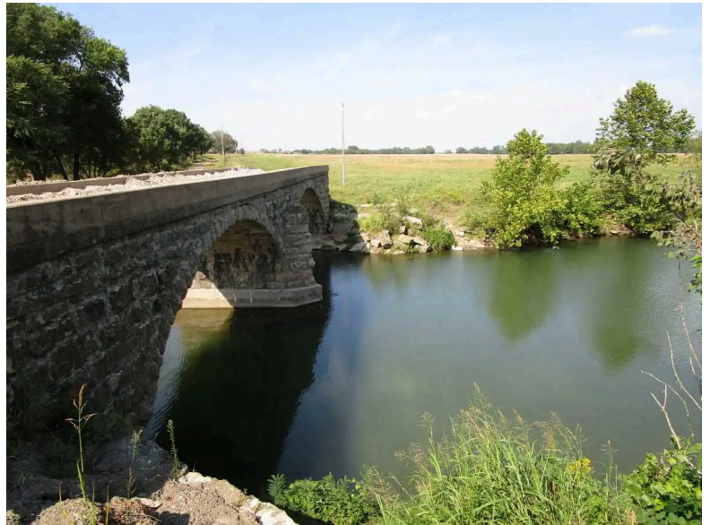
Stone Arch Bridge In Cowley County
